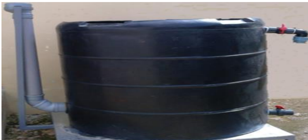
Figure 4. Placement of the outer tank on the metal base
