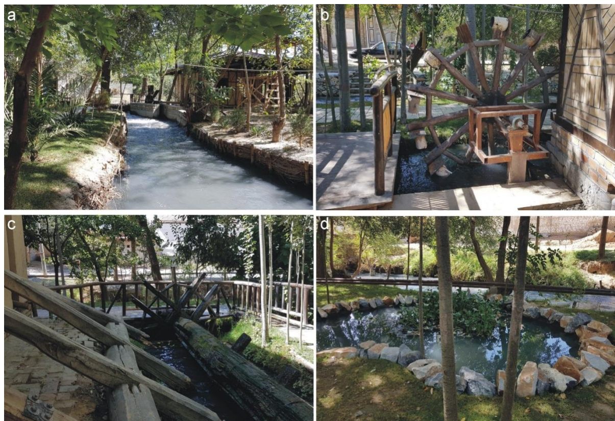
Figure 4. Small hydraulic structures in a mulberry paper factory: a – ditch bringing water to the factory; b – water wheel; c – grinder driven by the energy of flowing water; d – small pond.
